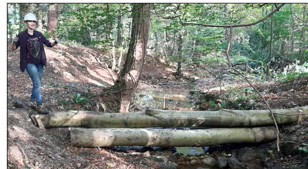
Leaky dams in Limb Brook © Rob Jones
